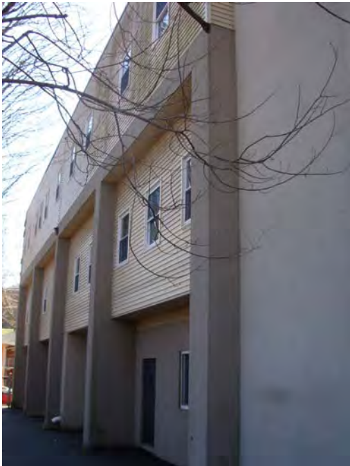
3. View of side-rear of building, note vinyl siding and EIFS
