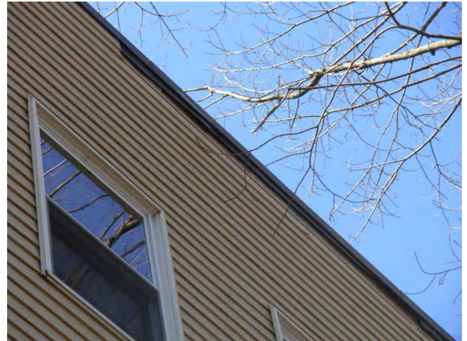
4. Spot vinyl siding damage and organic material growth
